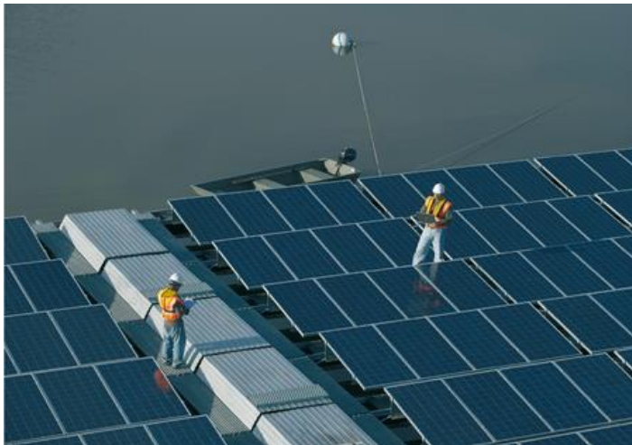
Figure 5. Napa Valley Winery 1.2MW System Example
